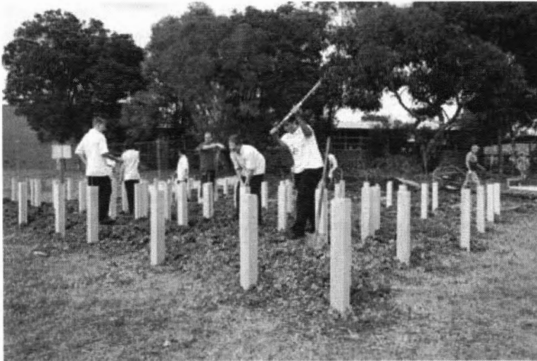
Figure 6: Students working on the foundations of the recording studio 18
