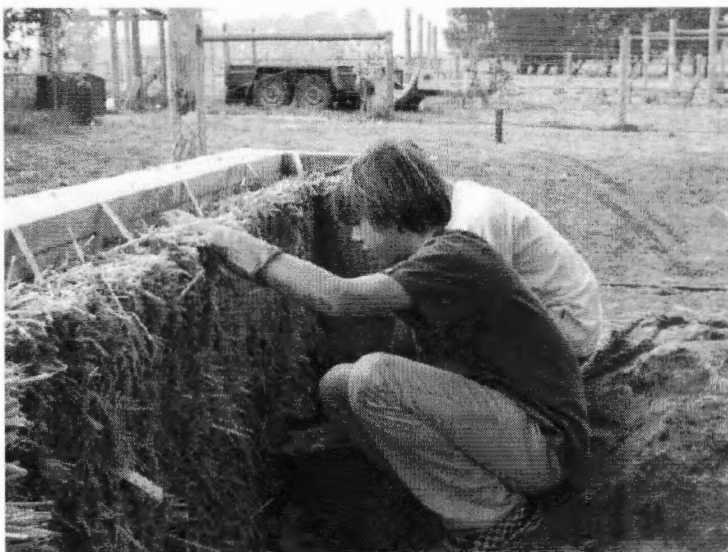
Figure 1: Woodleigh students constructing the straw bale walls (Source: Woodleigh School)
